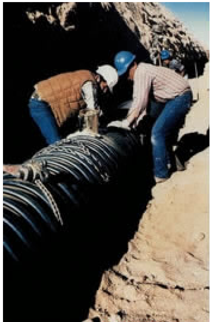
Assembling a Spirolite ® Joint
